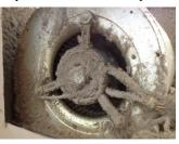
so dirty, the airflow has pulled the filter into the blower compart-
