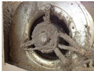
or if your filter is so dirty, the air-flow has p u l l e d the filter into the b l o w e r compartment and is drawing air from AROUND the filter. Don't let this be you.
